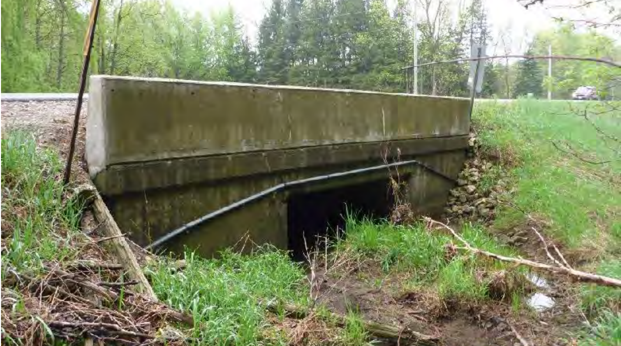
(S2) Structure 004-0901 Culvert 501 – West Elevation
