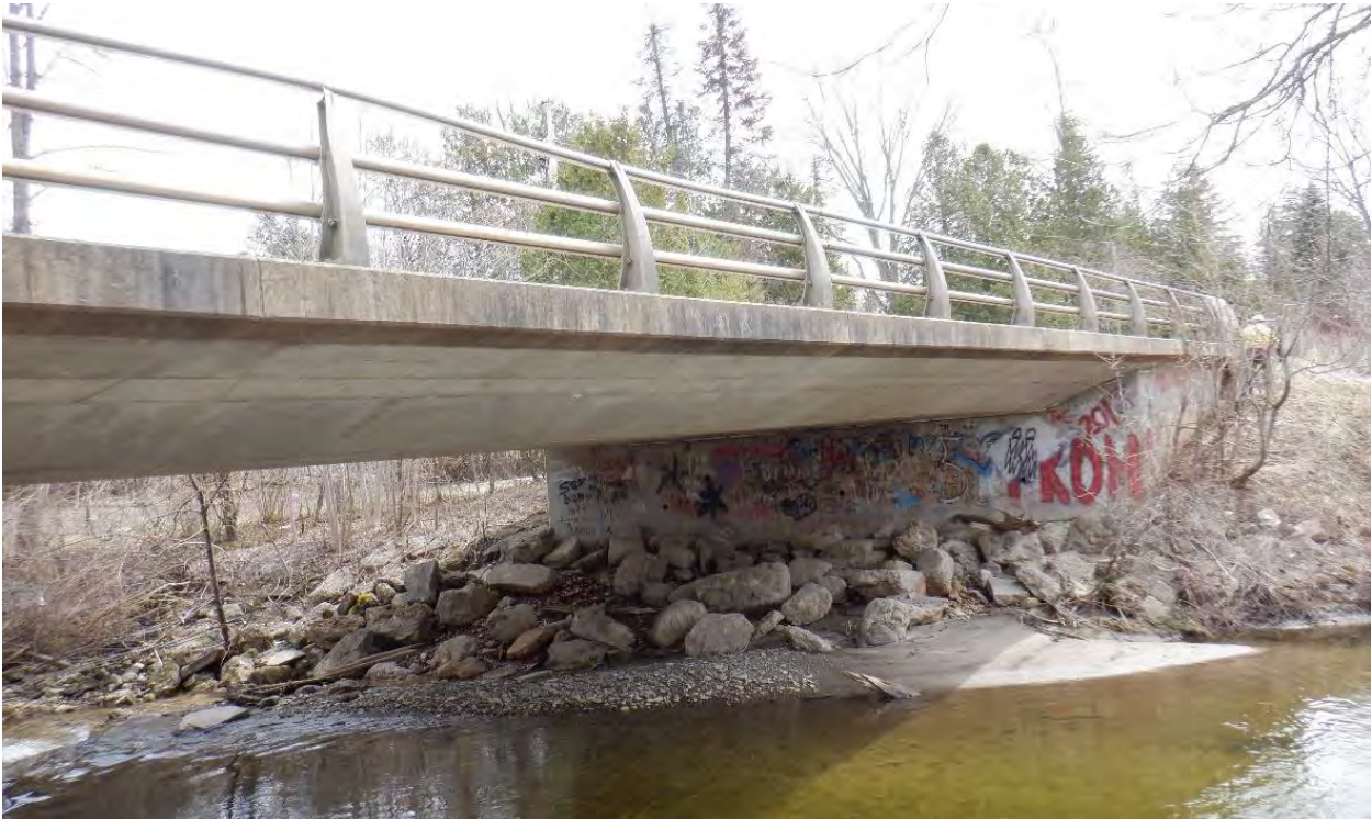
(S3) Structure 030-0318 Nottawasaga Bridge – Pre-Construction North Elevation
