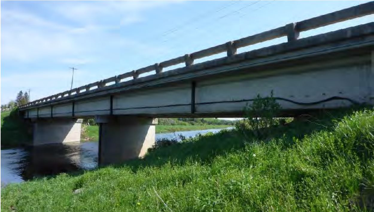
(S1) Structure 004-0142 Bridge No. 1 – West Elevation
