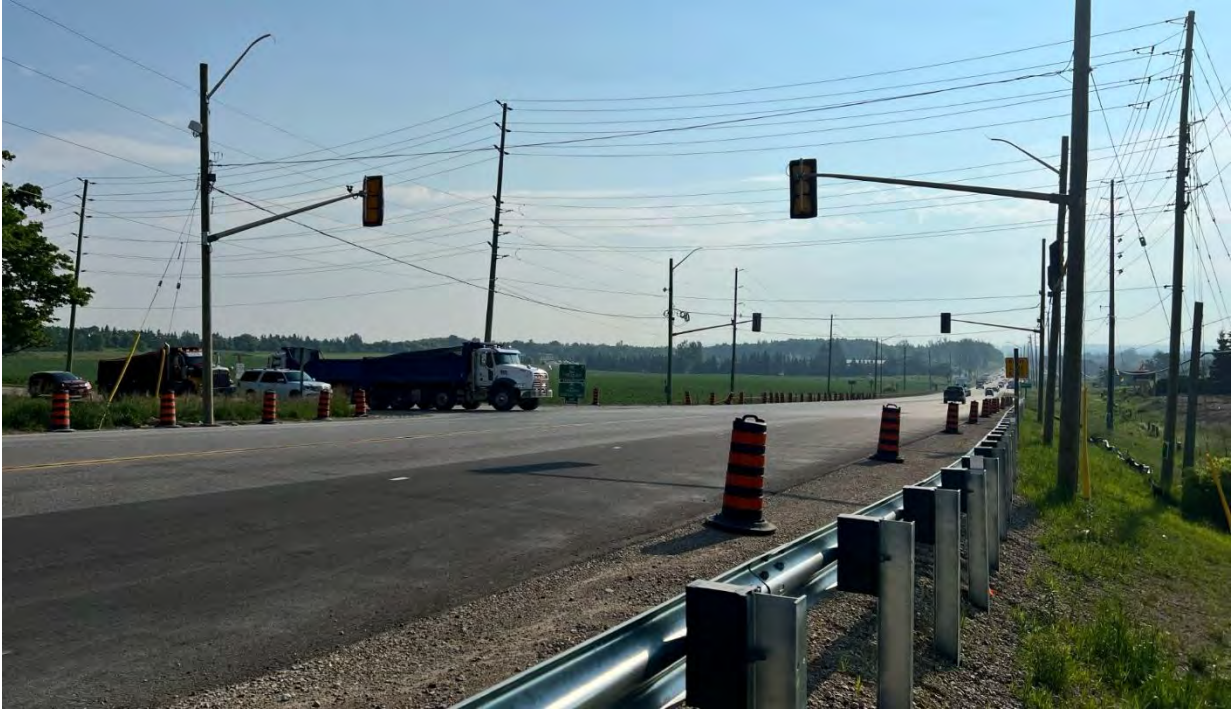
(R3) Dufferin County Road 109 at 2 nd Line Intersection – New Traffic Signal Lights
