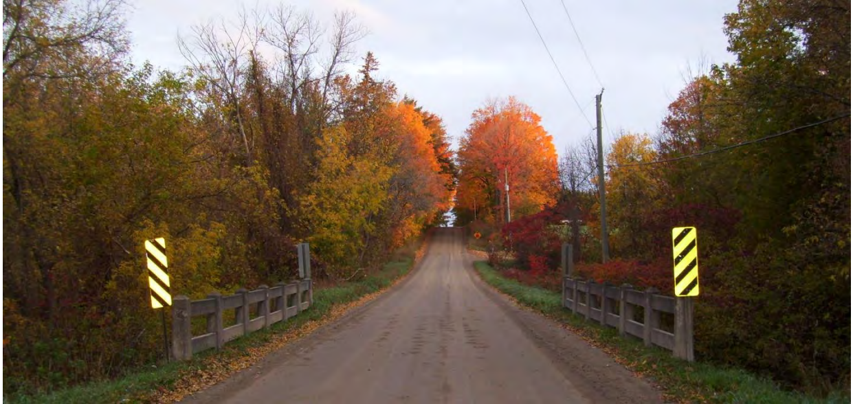
(S4) Structure 004-0007 Walkers Creek Bridge – Looking North at Bridge
