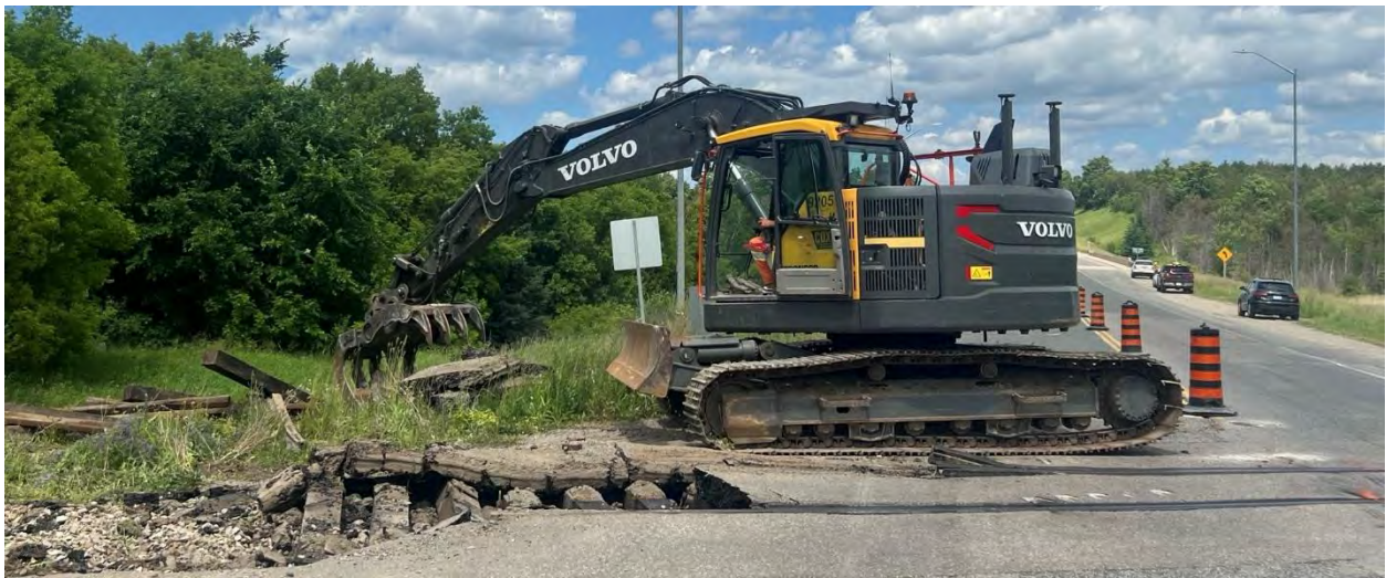
(R2) Dufferin County Road 109 South Arterial Road – Railway Crossing Removal
