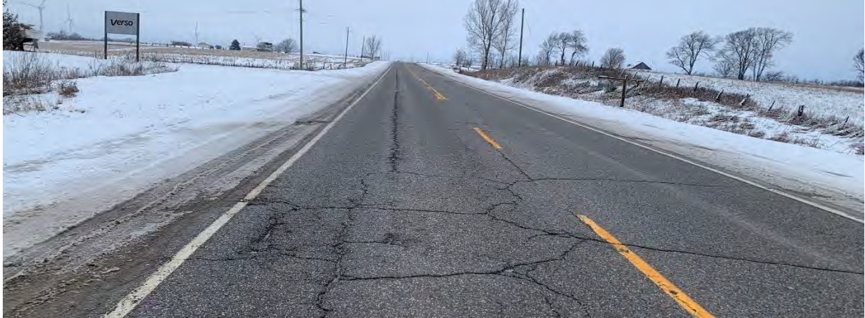
(R1) Dufferin County Road 124 – Pre-Construction Photo
